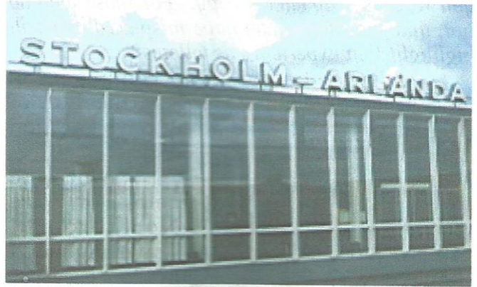
Stockholm's Arlanda Airport Terminal
